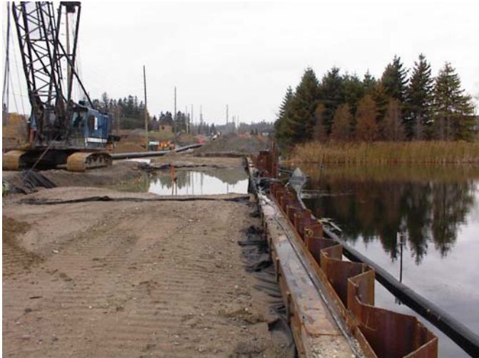
Photo 8: Pile driving in the McKenzie Wetland in the background. Sub-excavation and the placing of granular backfill in the foreground. Note the condition of the wetland adjacent to the work area.
