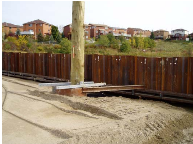
Photo 11: Temporary support of new hydro pole
