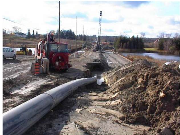
Photo 10: Installation of watermain under the road platform within the wetland using horizontal directional drilling.
