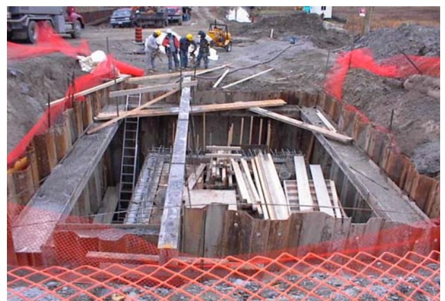
Photo 9: Construction of a sanitary sewer chamber around the existing sewer to complete the connections
