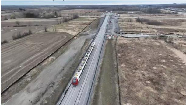
Figure 16 Embankment currently under active use (dynamic rolling stock testing)
