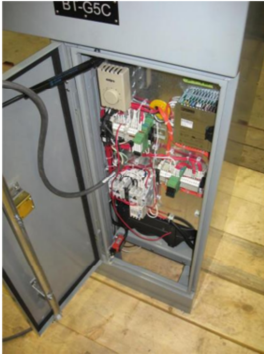
Figure 7 – Interior of Traffic Control Gate
