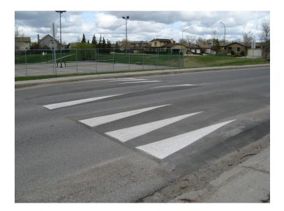
Figure 9 – Speed Cushion During Dry Conditions
