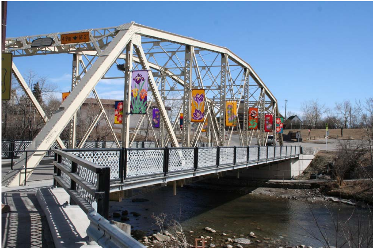
Photo 7: MacDonald Bridge Today
