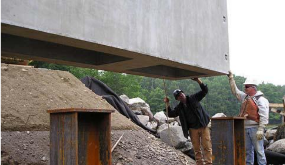
Figure 6: Placement of precast abutment section. (Source: PCI)
