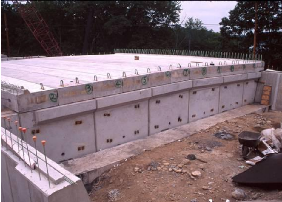
Figure 10: Completed integral precast abutment section. (Source: PCI)
