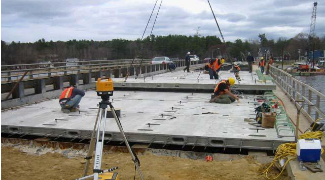
Figure 12: Placing precast deck slabs. (Source: PCI)
