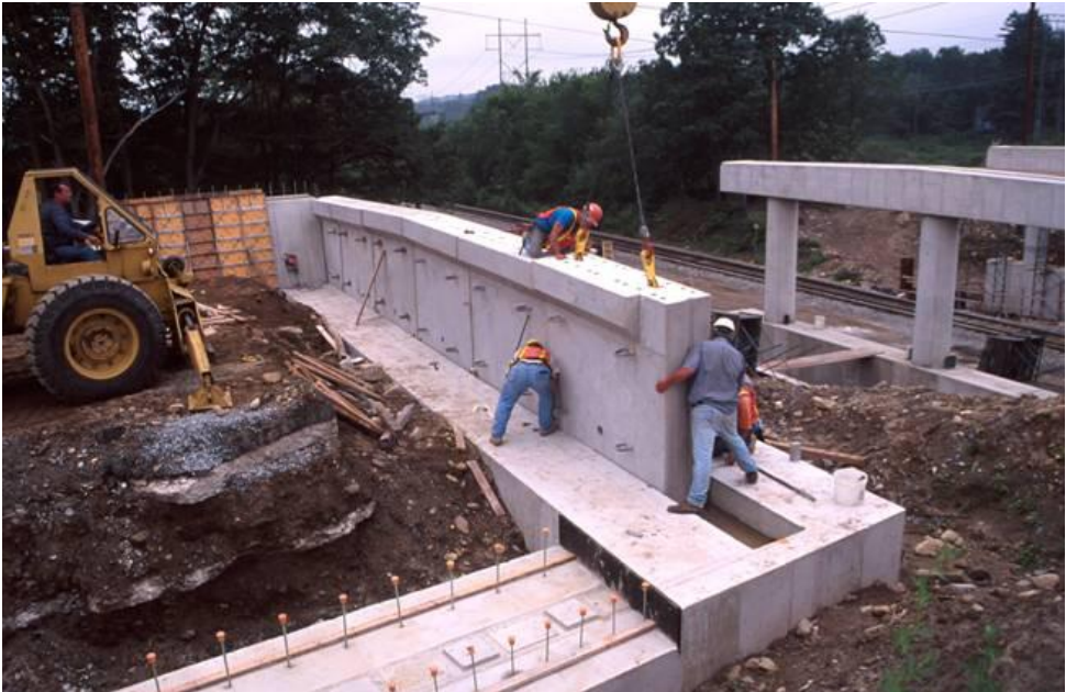
Figure 7: Precast abutment with pin connection. (Source: PCI)
