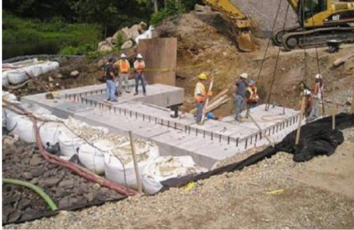
Figure 4: Completed segmental precast footing. (Source: PCI)
