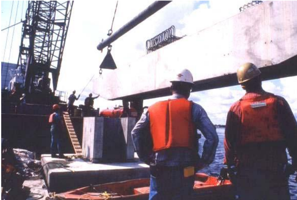
Figure 8: Assembly of a precast pier cap. (Source: PCI)
