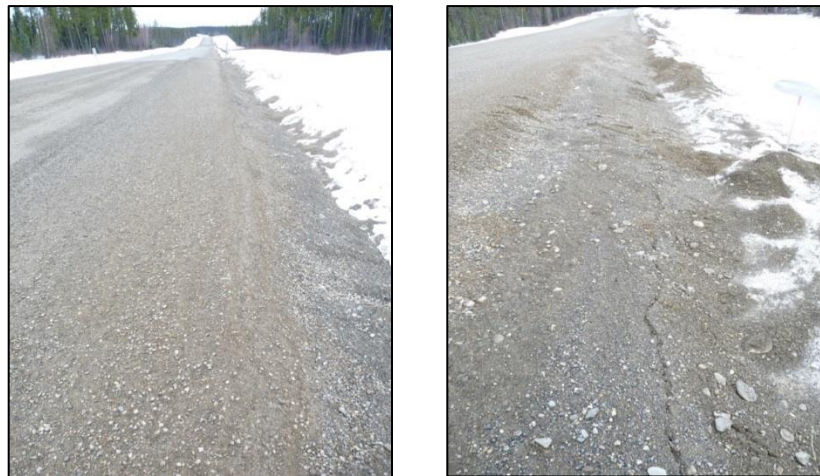
Figure 8. Edge cracking at site 6 looking south (left), and at site 4 looking north (right), spring 2016.
