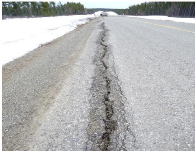
Figure 1. Edge cracking can be wide, deep and extensive.
