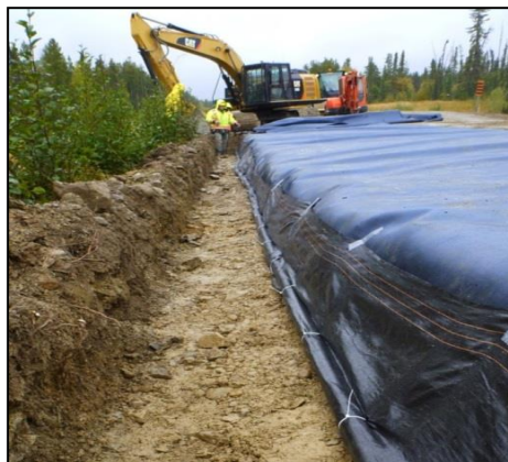
Figure 5. Mirafi® H2Ri edge in drain pipe hanging in trench at 1% slope
