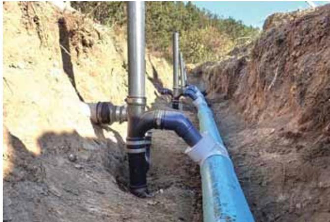
Figure 3-2: Installation of traps for housing conductivity sensors.
