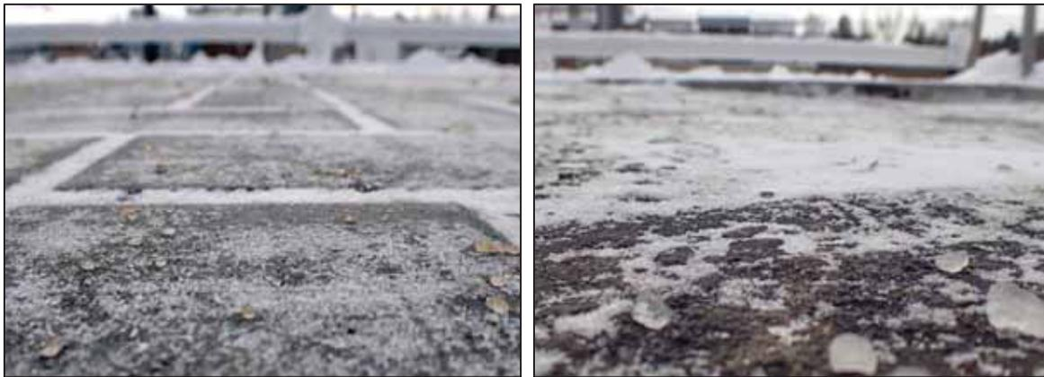
Figure 4-3: Comparison of pavement textures between PICP (left) and asphalt (right).
