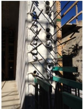
FIGURE 11 – AREA OF HIGH CONDUIT DENSITY IN TUNNEL WALL
