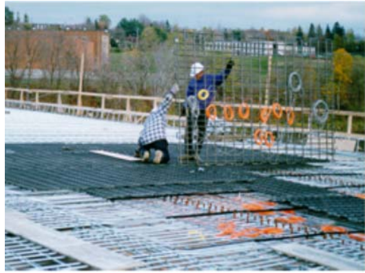
(b) Carbon FRP grids (Joffre Bridge)
