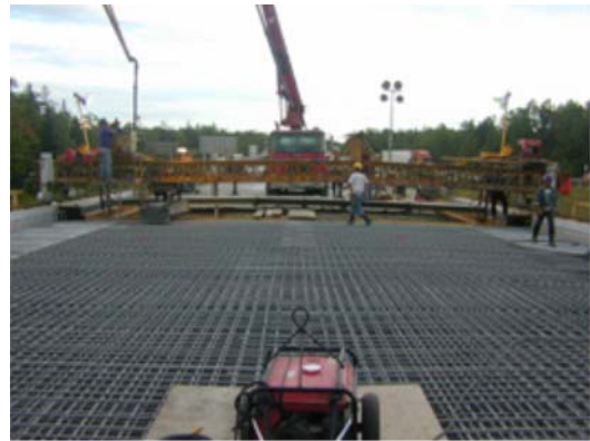
(f) FRP reinforcement for the deck slab (Magog Bridge)
