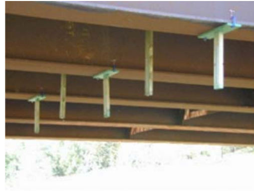
(b) Rulers installed on steel girders
