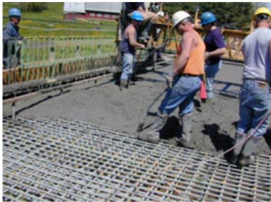
(e) Casting the bridge deck slab (Morristown Bridge)
