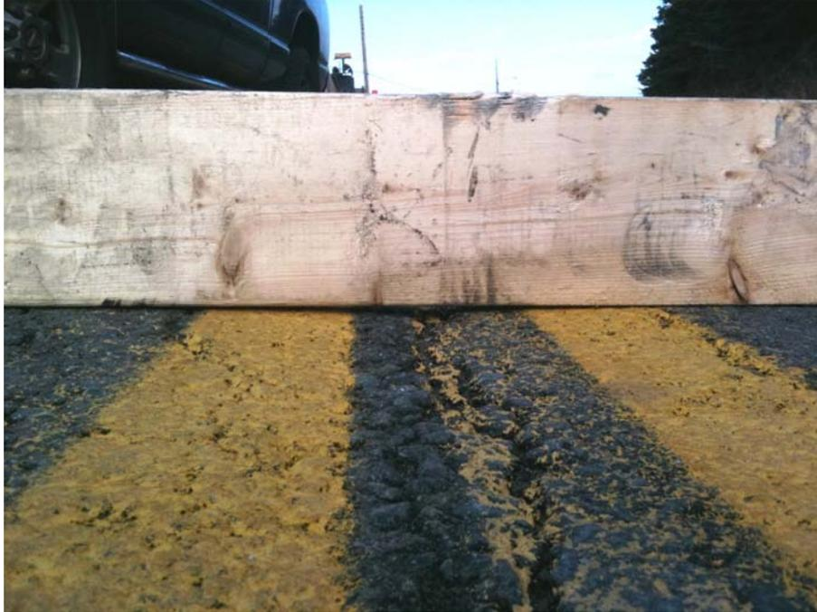
Figure 2 – Depressed crown in a region of moderate centreline cracking.
