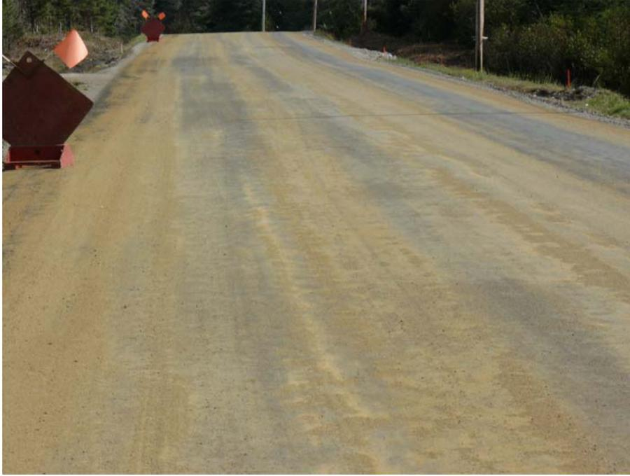
Figure 8 – Poor contact of micro-cracking effort on rutted surface of uncured PC-FDR mat.
