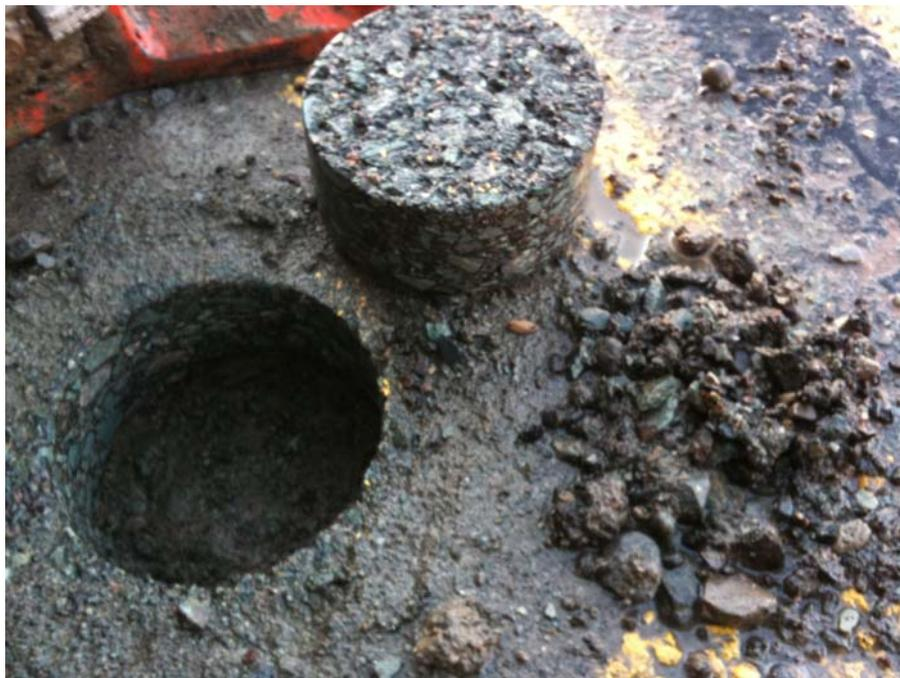
Figure 7 – Photograph of core location in heavily damaged PC-FDR base near the pavement centreline.
