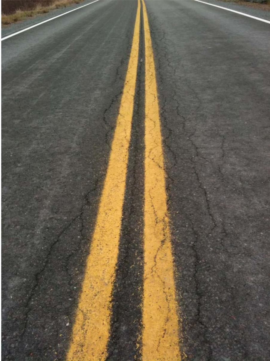
Figure 1 – Severe centreline cracking observed on Pt. Michaud beach Road PC-FDR pavement.
