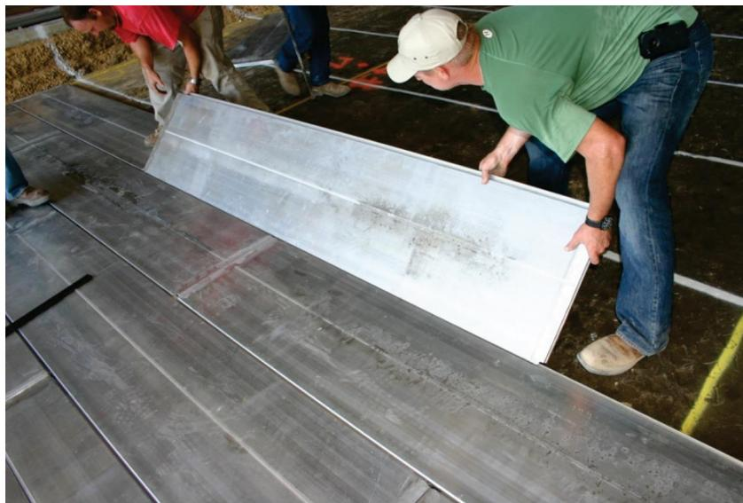
Figure 1: Installation of aluminum truss matting system S45 (Garcia, 2016).
