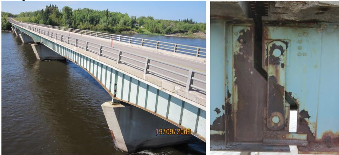
Figure 1 – View of the pre-rehabilitated bridge (left) and the pin-hanger system (right)
