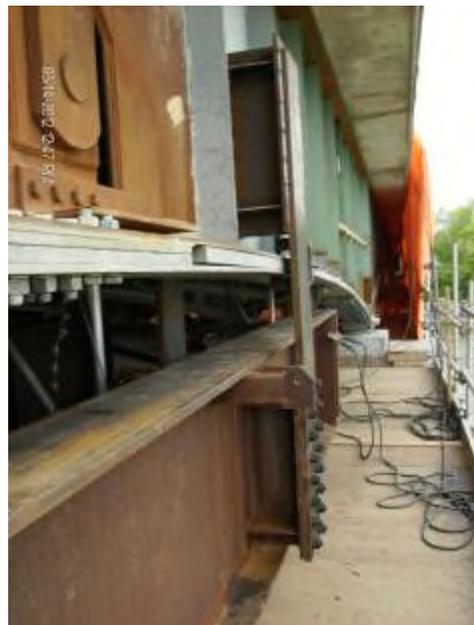
Figure 4 - Temporary Support System
