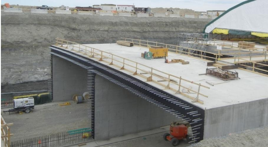
**Figure 4. Constructed Movement Joint**
