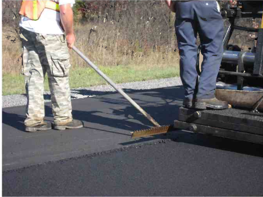
Figure 6 Photograph of WMA Joint Construction
