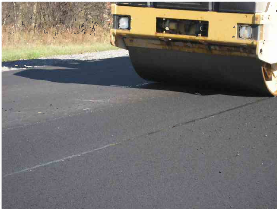
Figure 7 Compacting the Longitudinal Joint
