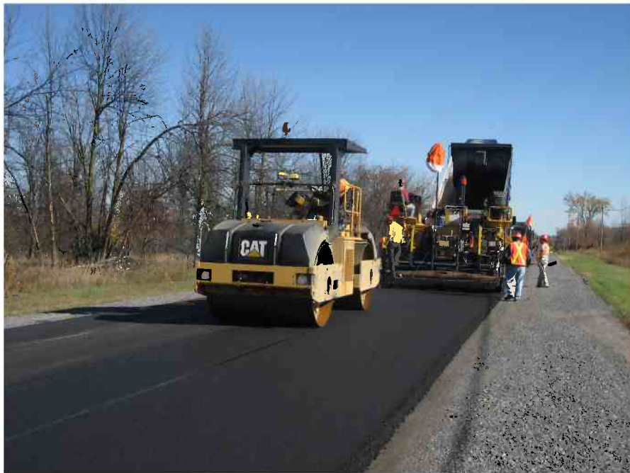
Figure 5 – Photograph of Paving and Breakdown Compaction
