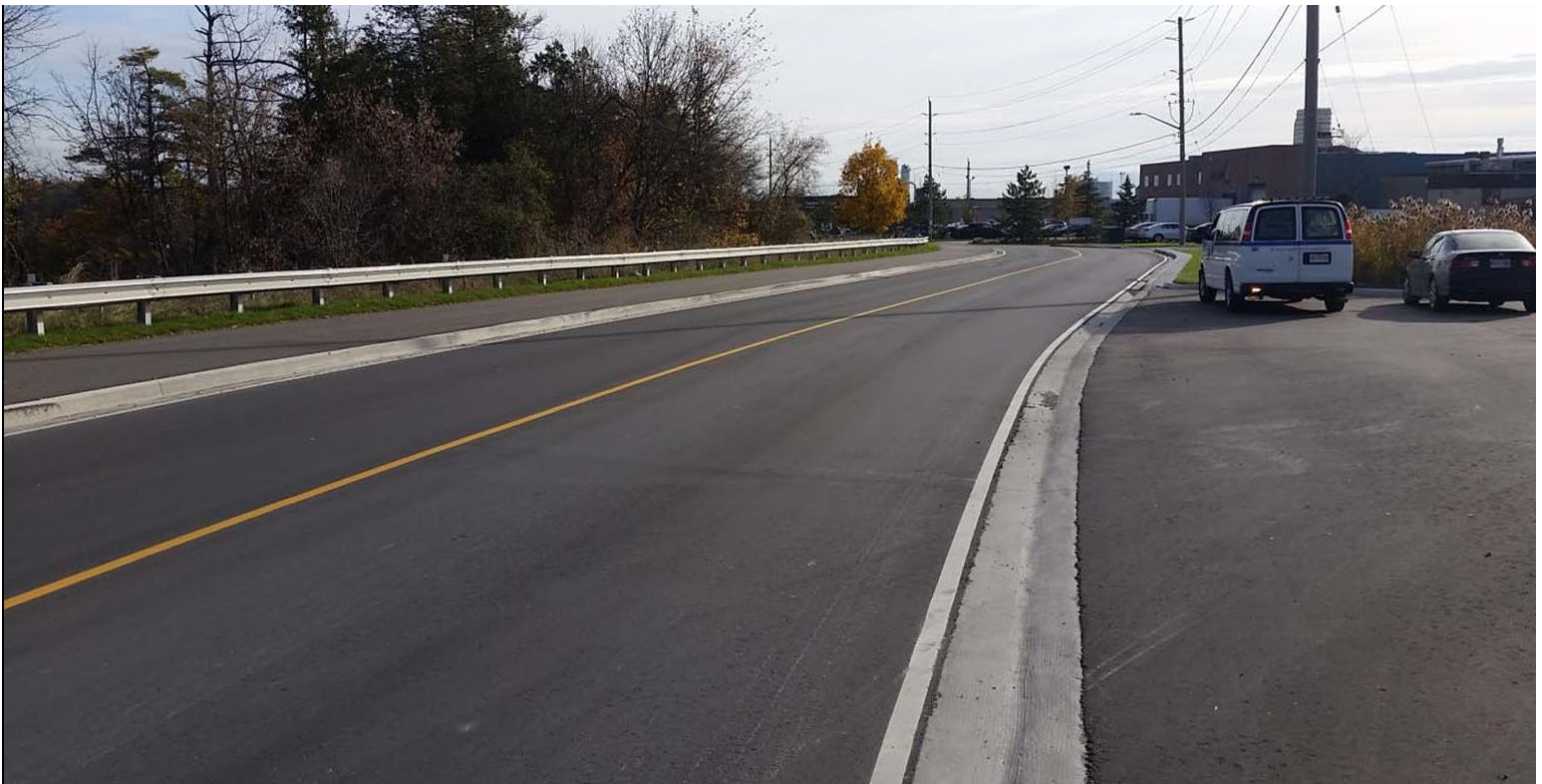
Armstrong Avenue – After Construction
