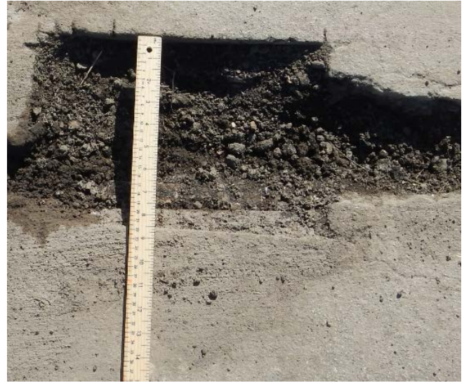
Figure 15: Moderate Pothole
