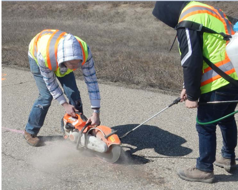
Figure 5: Fabricating Cracks using a Pavement Saw
