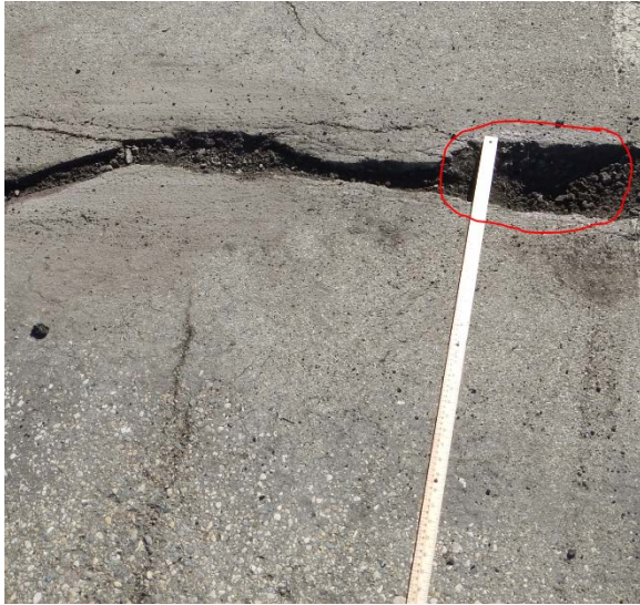
Figure14: Severe Pothole
