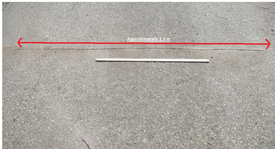
Figure 7: Testing Minimum Transverse Crack Length
