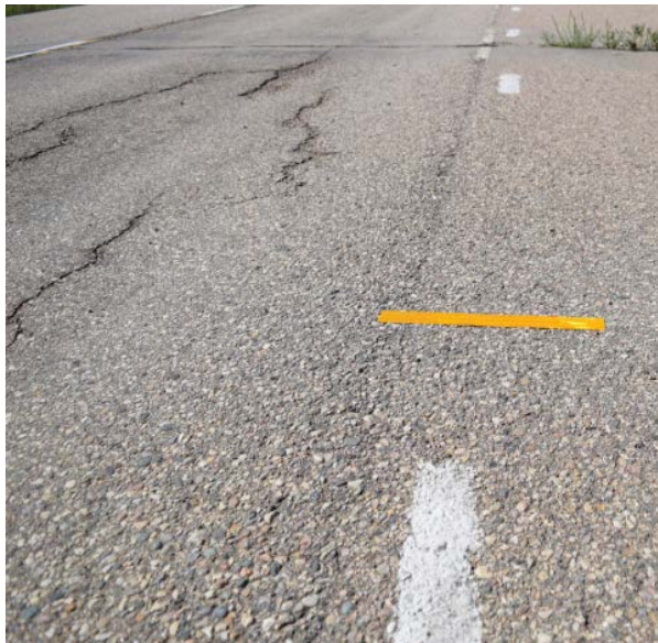
Figure 4: Lane Markings & In situ Cracking
