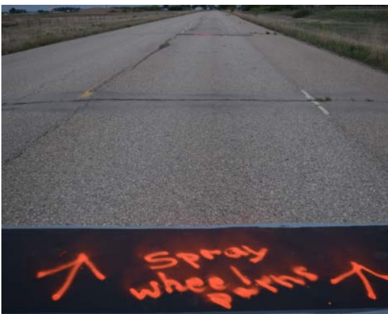
Figure 16: Construction Paper used to mask off Bleeding Area
