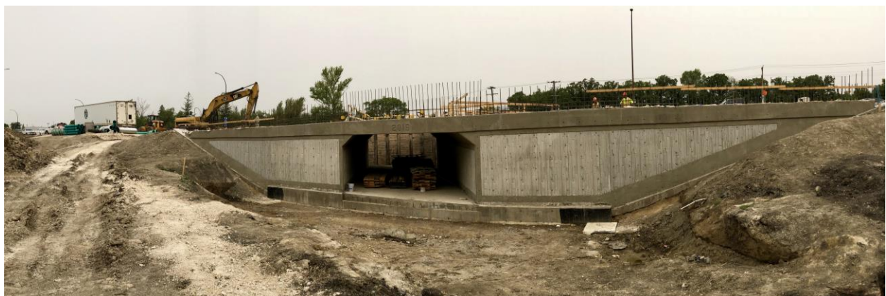
Figure 14 – Pedestrian-Cyclist Underpass Under Construction
