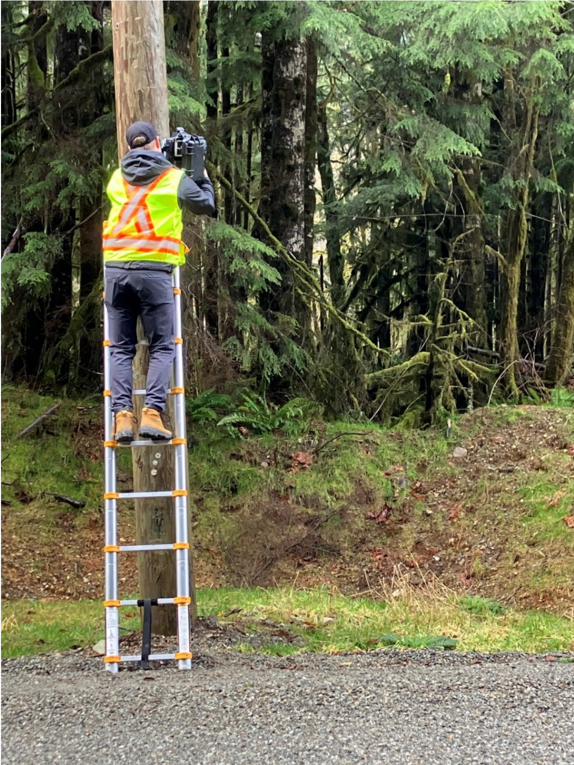
Figure 3: MOTI staff member installing traffic radar system on utility pole
