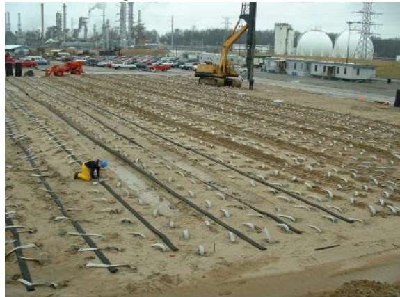
Figure 8. Vertical Drains
