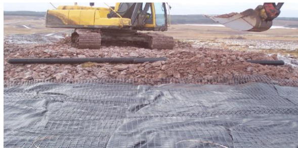
Figure 10. Geotextile reinforcement
