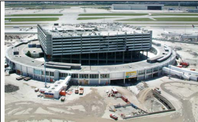
Figure 1: Old Terminal One – Demolition on Level 9 (June 25, 04)
