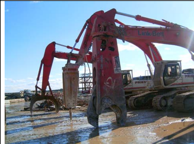
Figure 3: Demolition Equipment – Shear (right), Pneumatic Hammer and Grapple (left)
