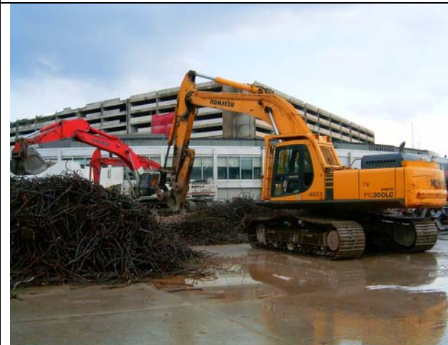
Figure 9: Rebar Scrap being processed
