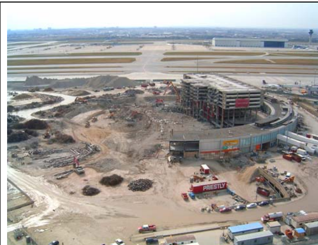
Figure 7: Demolition Site – Stockpiled Salvaged Material around Old T1
