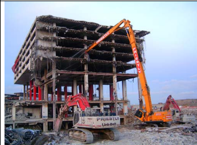
Figure 5: Demolition Equipment – Shear (left), Pneumatic Hammer and Grapple (right)
