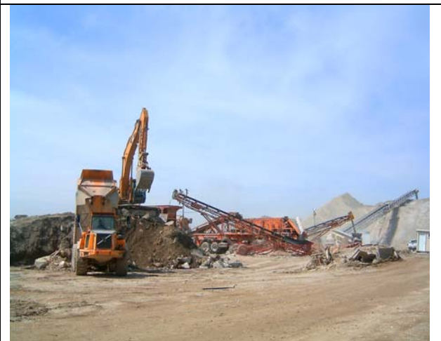
Figure 11: Concrete Crushing Plant and Processed Concrete Backfill
