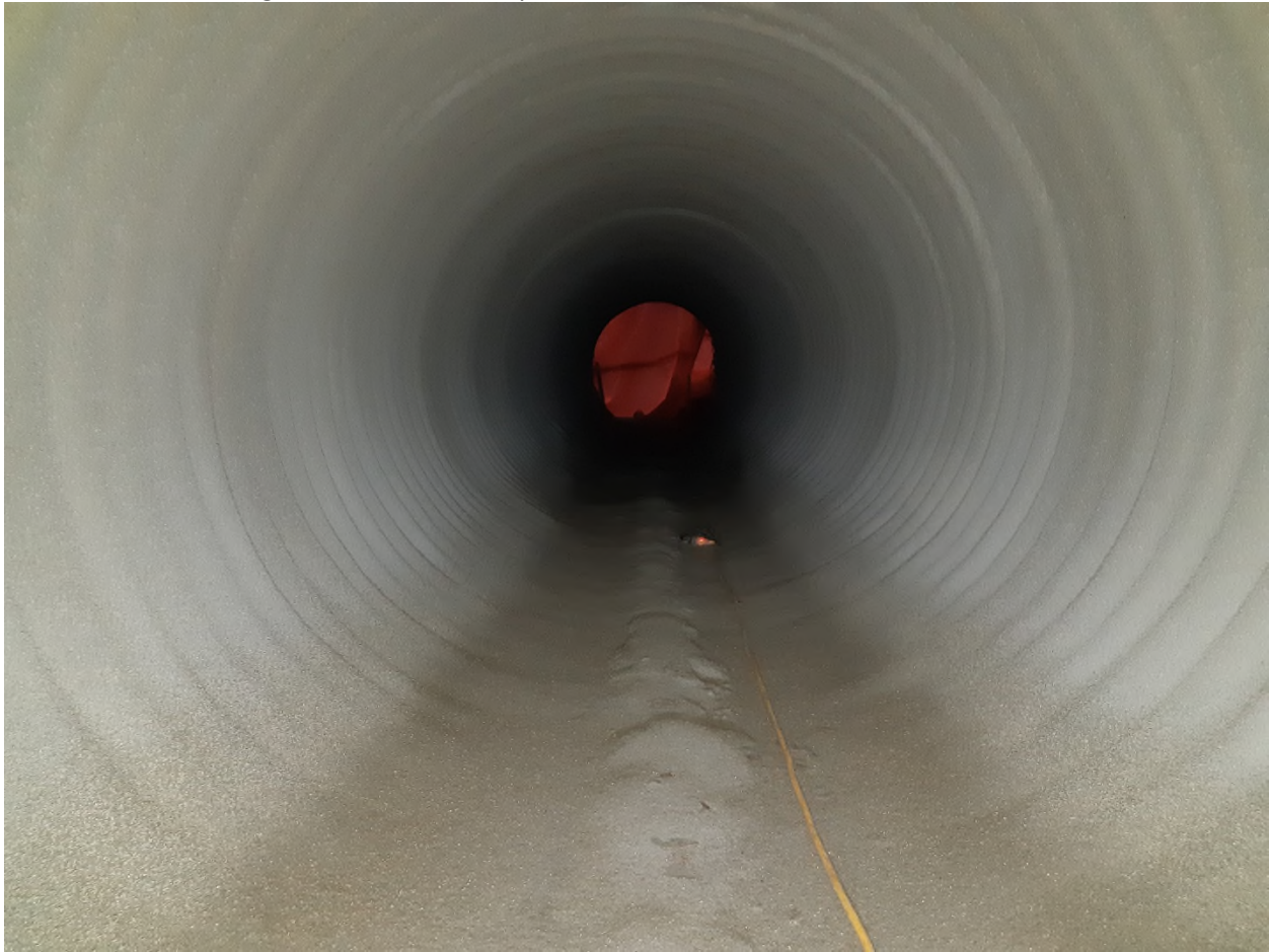
Figure 4. QC17 - Invert protrusion above location of ABS diversion
