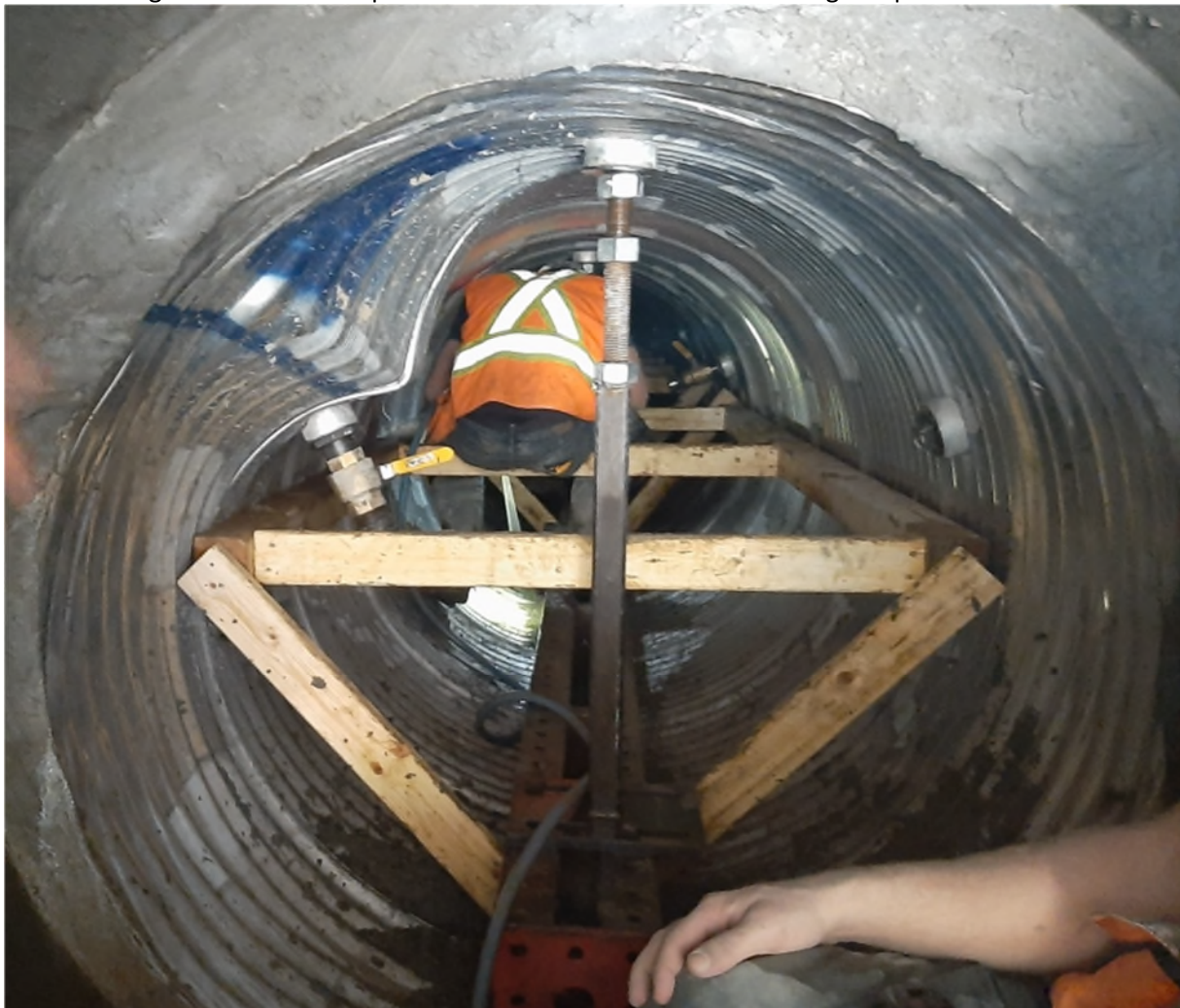
Figure 5. YT16 - Collapse of CAP Section due to Over Grouting – September 2021
