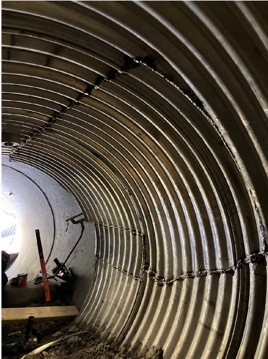
Figure 6 – YT16 - Repaired CAP - October 2021
