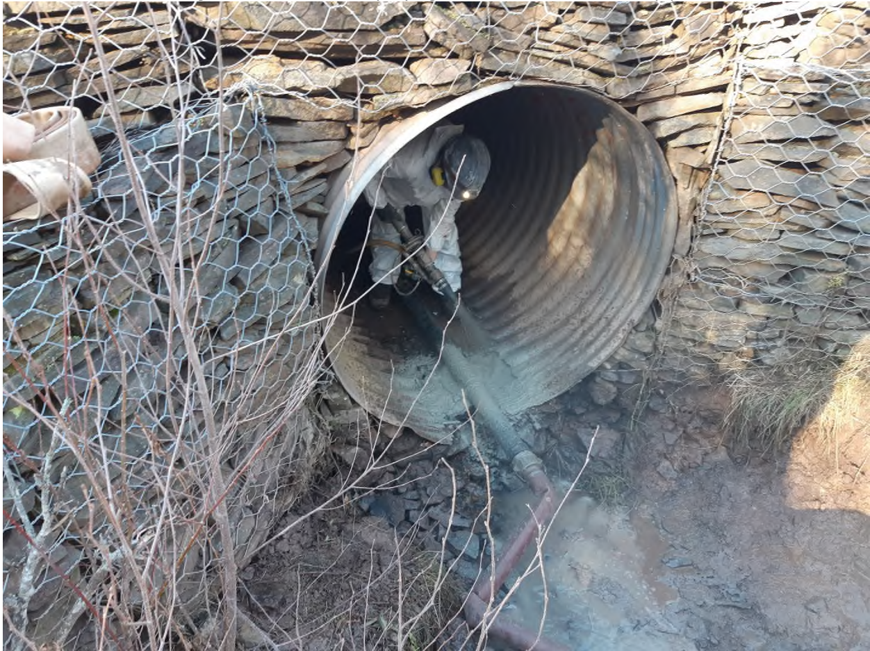
Figure 3. QC17 - Hand spraying over ABS water diversion pipe
