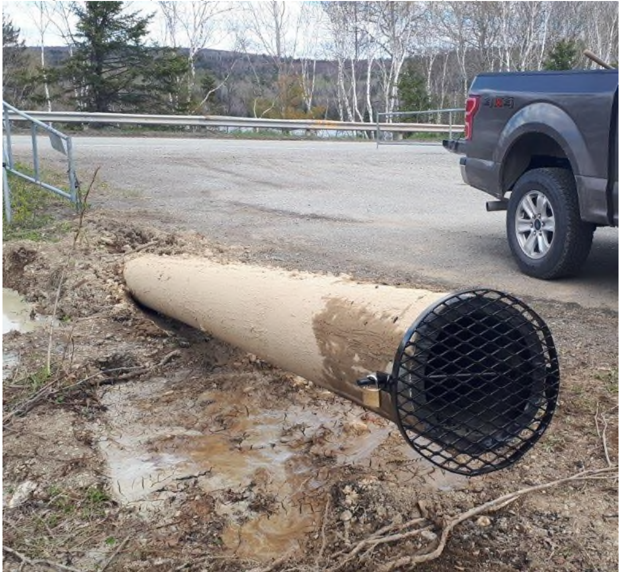
Figure 2. YT16 – Pipe Casing Installed by Directional Drilling for Temporary Water Diversion
