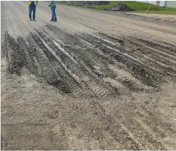
Figure 3: Rut depth before subbase preparation
