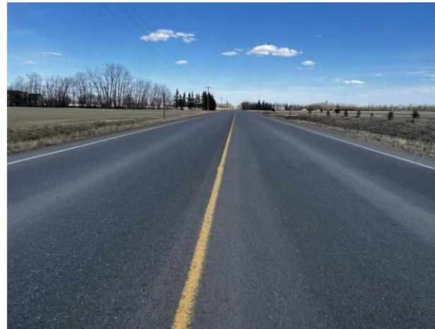
Figure 20: Current road condition at 100mm geocell section
