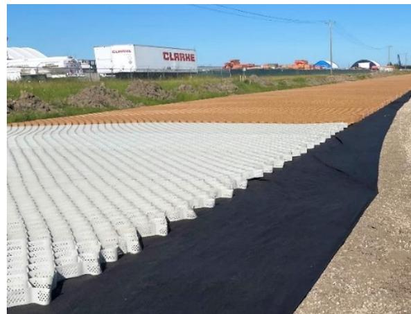
Figure 16: Basecourse fill over 150mm geocell and Combigrid sections
