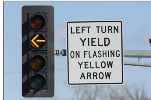
Figure 6: Supplemental Sign for FYA Signal installed in Minnesota
