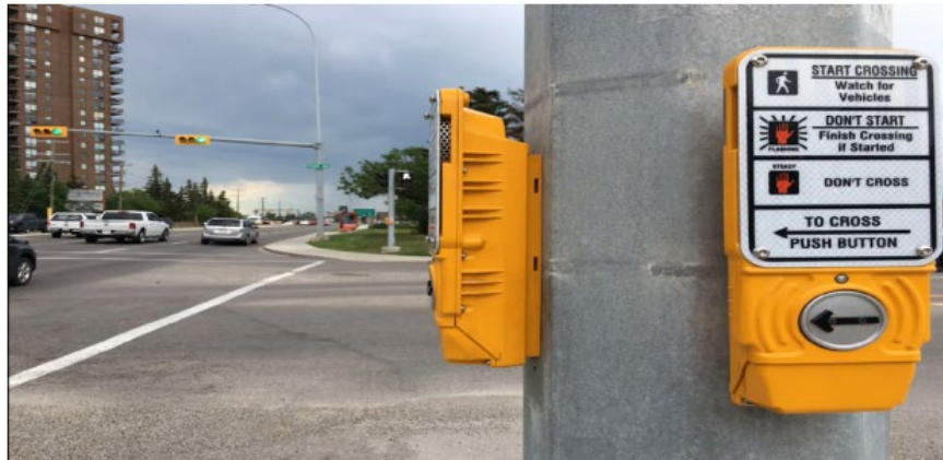
Figure 2-18: Accessible Pedestrian Signals (APS)
