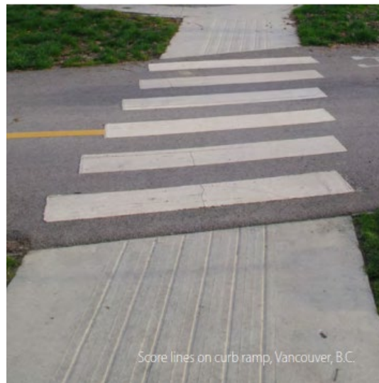
Figure 2-19: Score Lines on Curb Ramps
