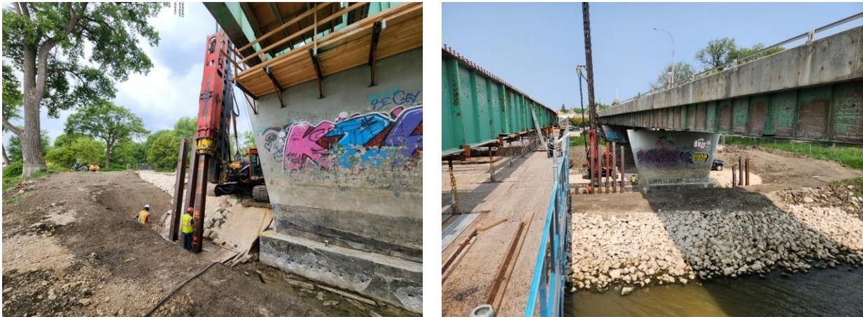
4. The piles were cutoff to the desired embedment into the new encasement pile cap. A working base slab was placed surrounding the existing pile cap to allow for assembly of the reinforcing steel cage around the piles, as shown in Figure 17. The working base slab further allowed the contractor to control seepage from the river, which was near the same elevation as the excavation base.
