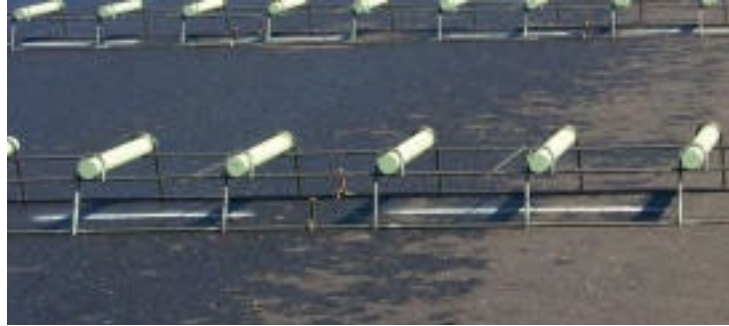
Figure 2: Dowel Basket Assembly
