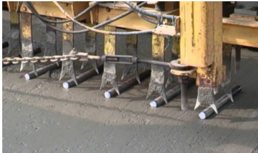
Figure 3: Dowel Bar Inserter on Slipform Paver
