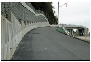
Figure 26 - Tiered and Stacked Retaining Wall (RW87)
