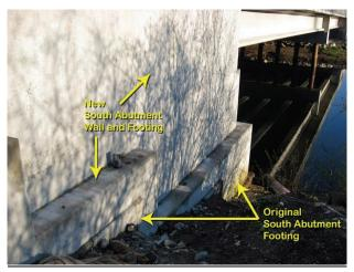
Figure 9 – Reuse of South Abutment Footing
