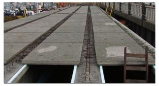
Figure 6 – Precast Concrete Deck Panels
