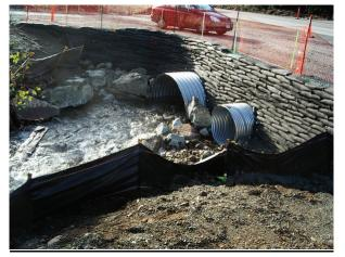
Figure 27 - Deltalok Wall Before Vegetation (Dryden Creek Culvert, Inlet Headwall)
