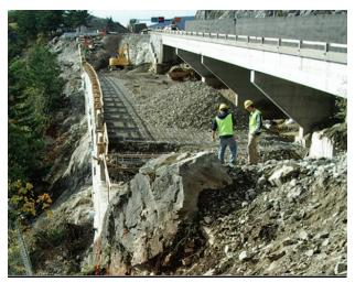
Figure 24 - MSE Wall Construction (RW993)
