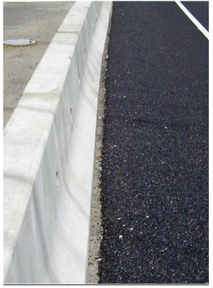
Figure 29 – Longitudinal Drainage Channel in Front of Concrete Barrier
