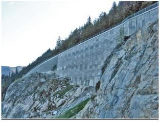
Figure 23 - Completed Hybrid Retaining Wall (RW1025)
