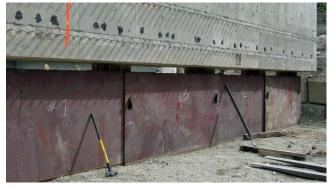
Figure 17 – Backfill Side of Steel Scour Protection Plates
