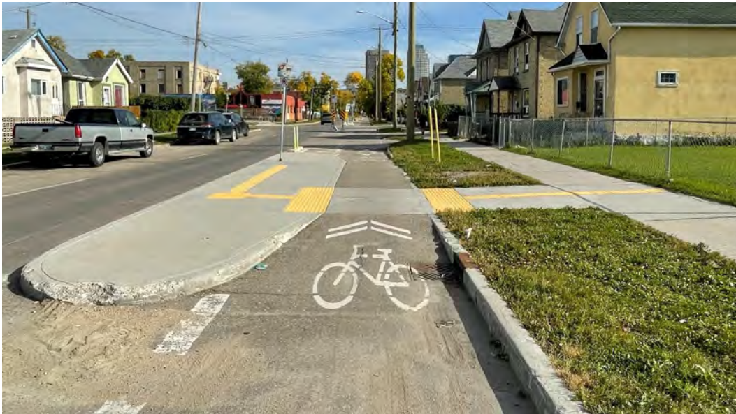
Figure 3: Island platform bus stop on McDermot Avenue in Winnipeg
