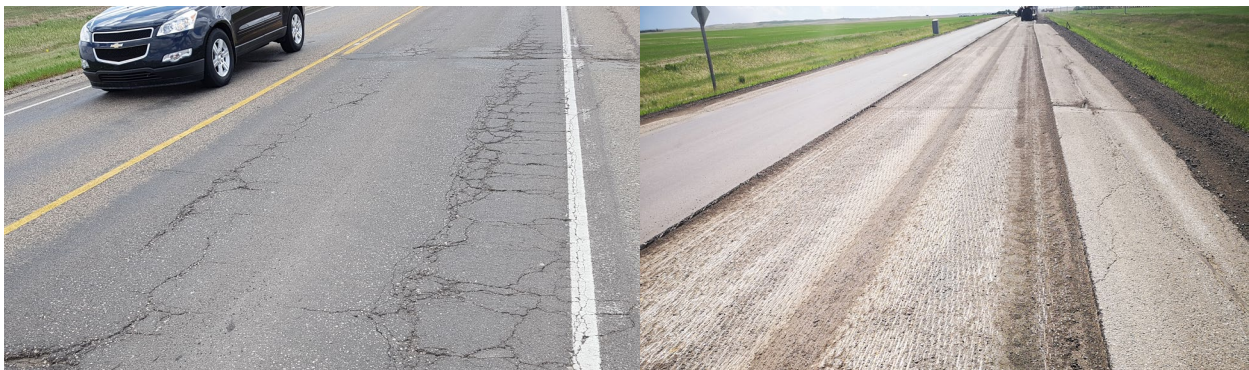
Figure 4. Highway 7 150-200A+HL Test Section, Pre- and Post-Milling
