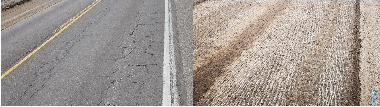
Figure 5. Highway 7 PG 58-37P+HL Binder Test Section – Pre- and Post-Milling
