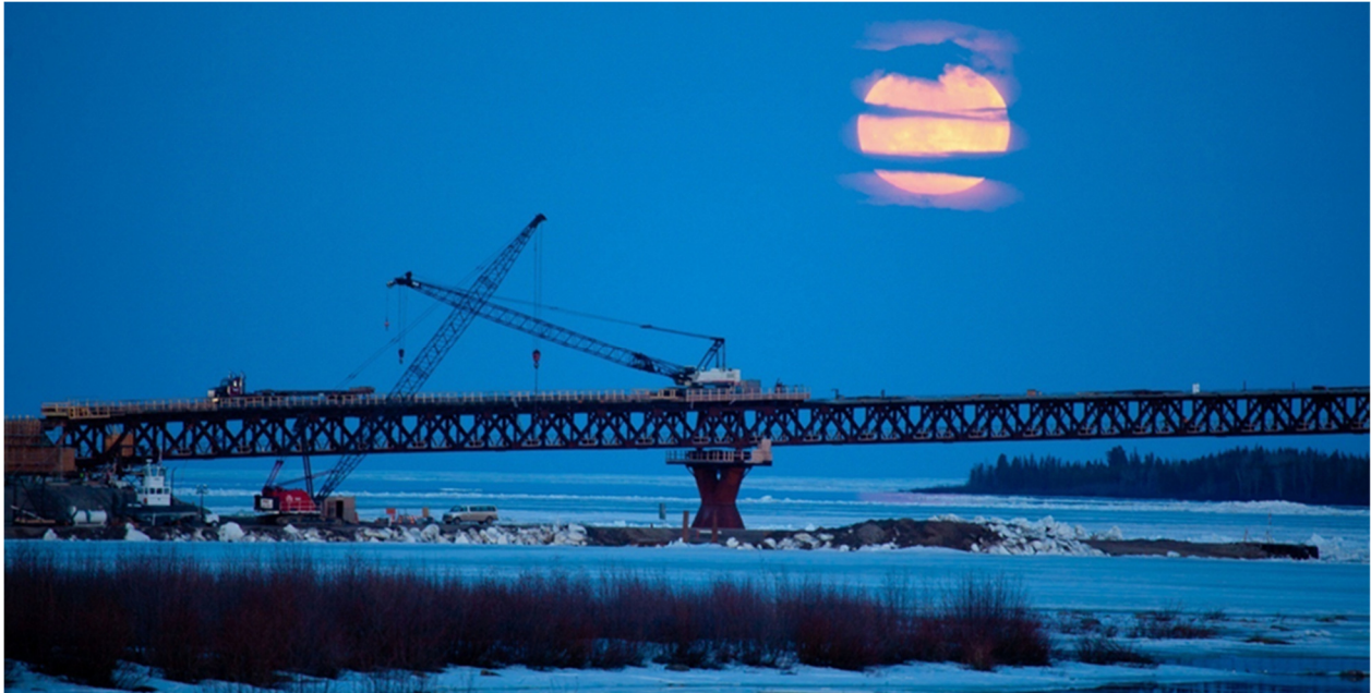
Figure 4. Deh Cho Bridge deck panel installation via work bridge placed on the truss
