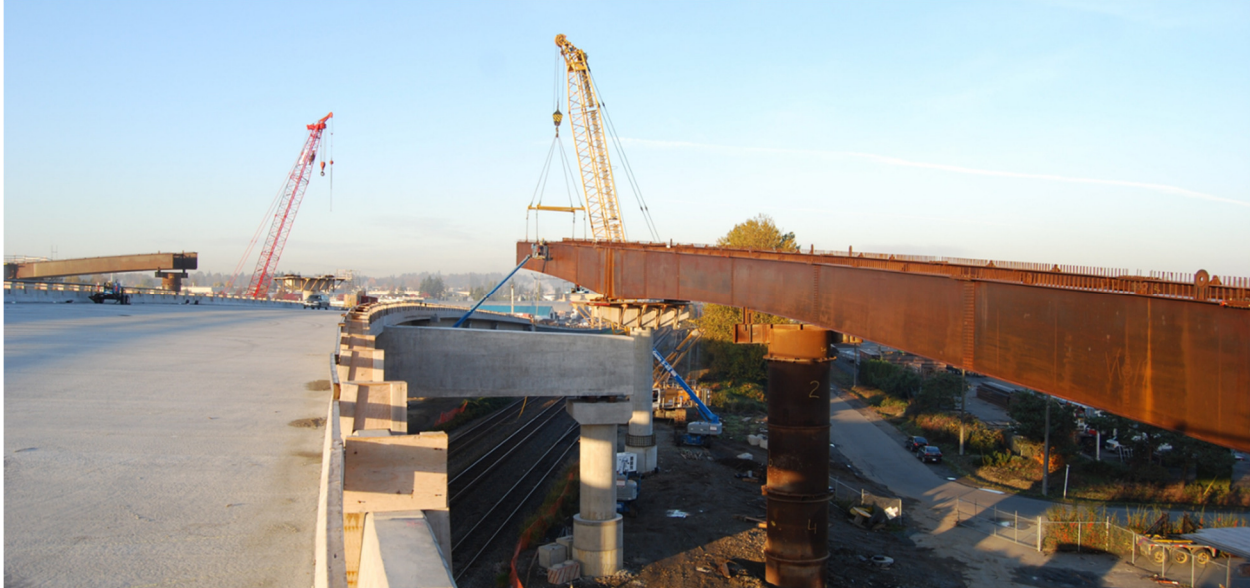
Figure 1. 199A Ramp superstructure erection via the progressive cantilever method
