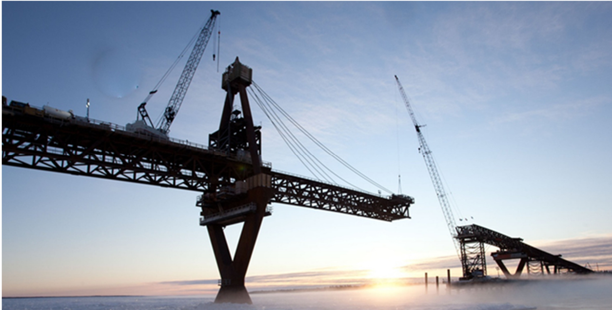
Figure 3. Deh Cho Bridge cable installation and superstructure launching
