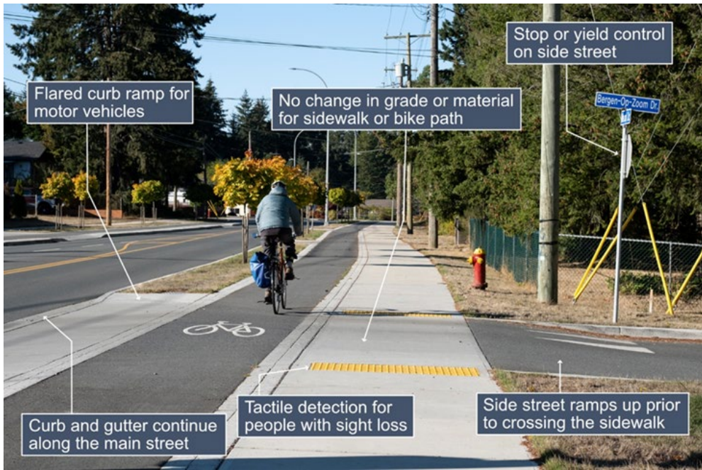
Figure 3: Basic features of a continuous sidewalk and bike path (Nanaimo, BC)
