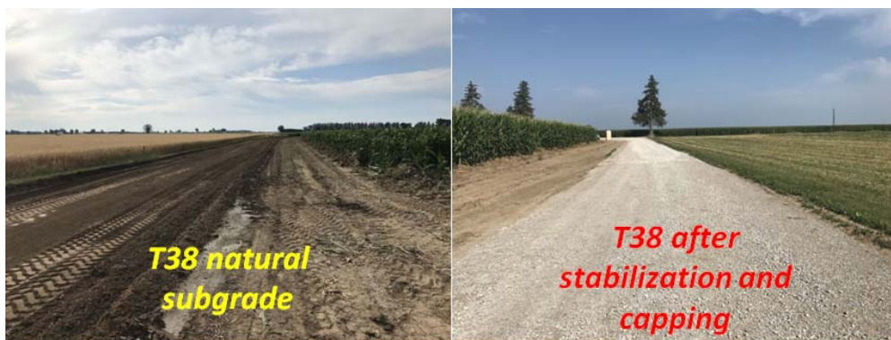
Figure 3. Road conditions: T38 before and after and construction, July 2017
