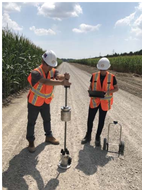
Figure 2. LWD test on T32, August 2017
