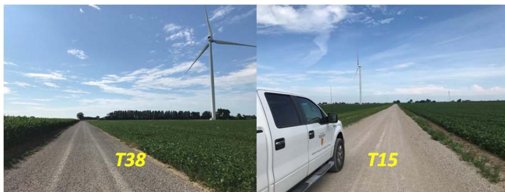
Figure 4. Road conditions: T38 (left) and T15 (right) after 1 year of construction, July 2018
