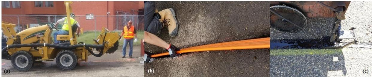
Figure 1: Micro-trenching Procedure. (a) Cutting the trench. (b) Laying cable. (c) Backfilling
