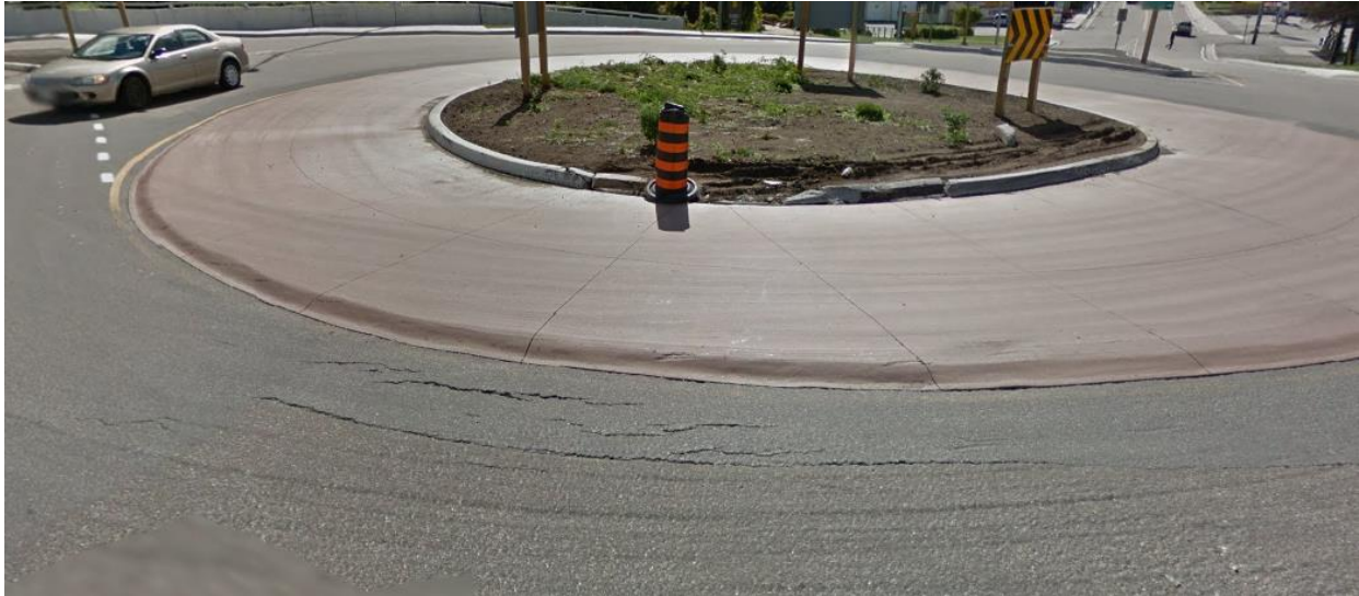
Figure 3. Example of distresses of asphalt pavement at a roundabout. Asphalt shoving, cracking and slippage are clearly visible.
