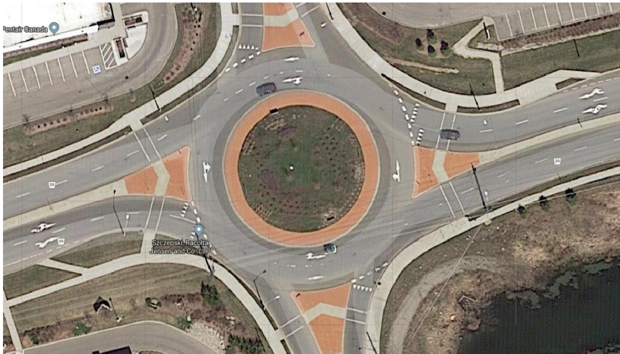
Figure 1. Roundabout constructed in the Regional Municipality of Waterloo in Ontario.
