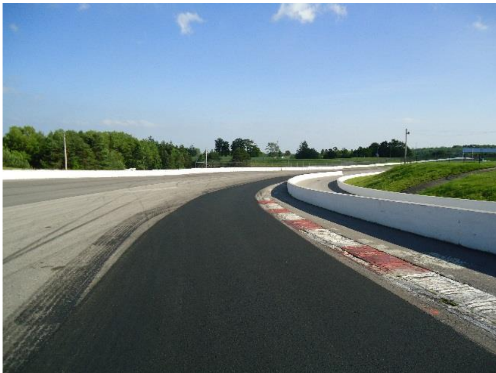
Figure 8. Advanced asphalt pavement placed on Mosport Race Track in 2013.
