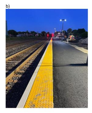
Figure 8 - Installation of a precast curb along the track.
