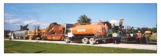
Figure 3. Cold-In-Place Recycled Expanded Asphalt Mix Train
