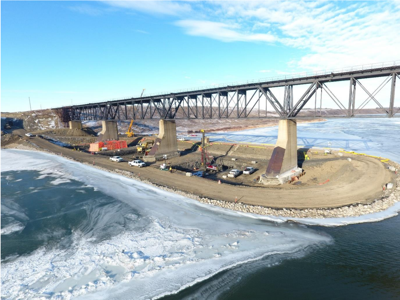
Figure 3 – Piling at Pier 7
