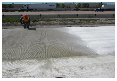
Figure 3. Concrete Pavement with Transverse Tining on Highway 401
