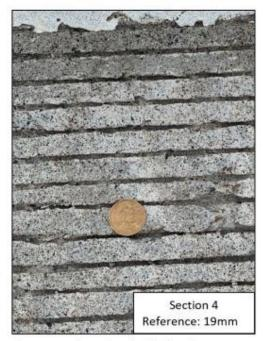
Concrete - Longitudinally tined
