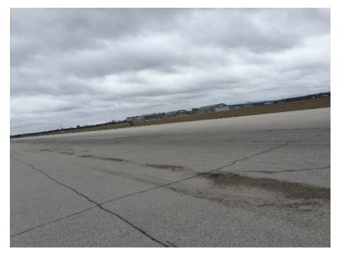
Photograph 11: Localized severe raveling on Runway 13-31.
