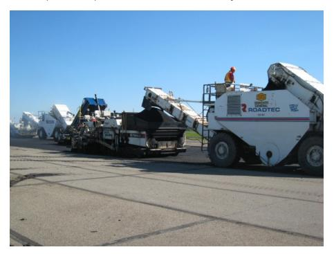
Photograph 8: Asphalt paving operation on Runway 02-20 included three pavers and two ShuttleBuggies<sup>®</sup>.
