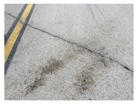
Photograph 13: Ravelling, cracking and polished aggregate.
