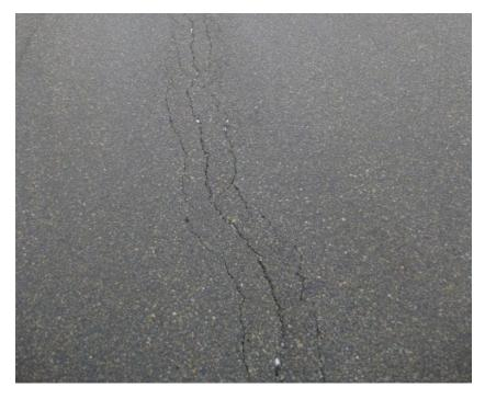
Photograph 3: High severity reflective cracking on the runway pavement.
