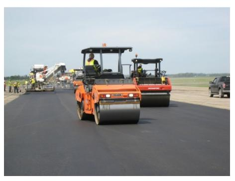
Photograph 9: Compaction operation on Runway 12-30.
