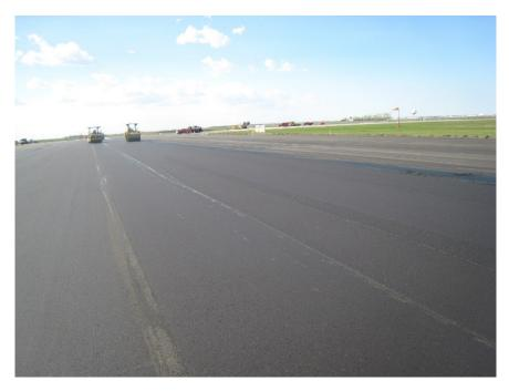
Photograph 19: Excellent quality of surface course mat. Longitudinal joint is very tight.
