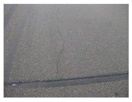
Photograph 2: Typical medium severity reflective cracking on the runway pavement.
