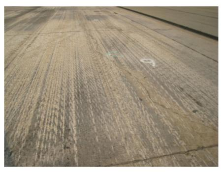
Photograph 6: Example of cross stitched crack in concrete slabs.
