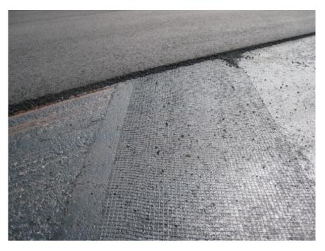
Photograph 17: GlasGrid® placed on existing pavement below the lower course.
