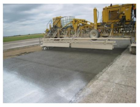
Photograph 5: Construction of new slabs on Runway 02-20.
