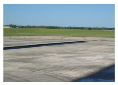
Photograph 7: Prepared surface of the concrete on Runway 12-30 prior to tack coat application and placement of new HMA.
