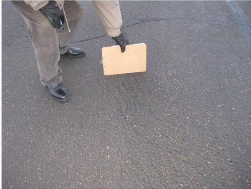
Photograph 4: Shear cracking and shoving of the asphalt surface at a threshold of Runway 12-30.
