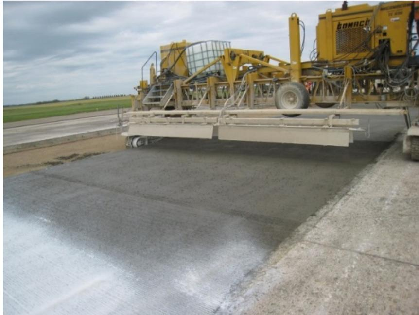
Photograph 5: Construction of new slabs on Runway 02-20.
