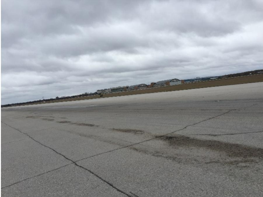
Photograph 11: Localized severe raveling on Runway 13-31.
