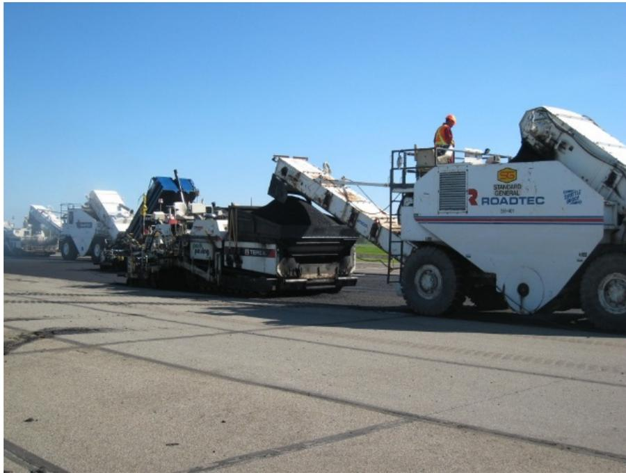
Photograph 8: Asphalt paving operation on Runway 02-20 included three pavers and two ShuttleBuggies®.
