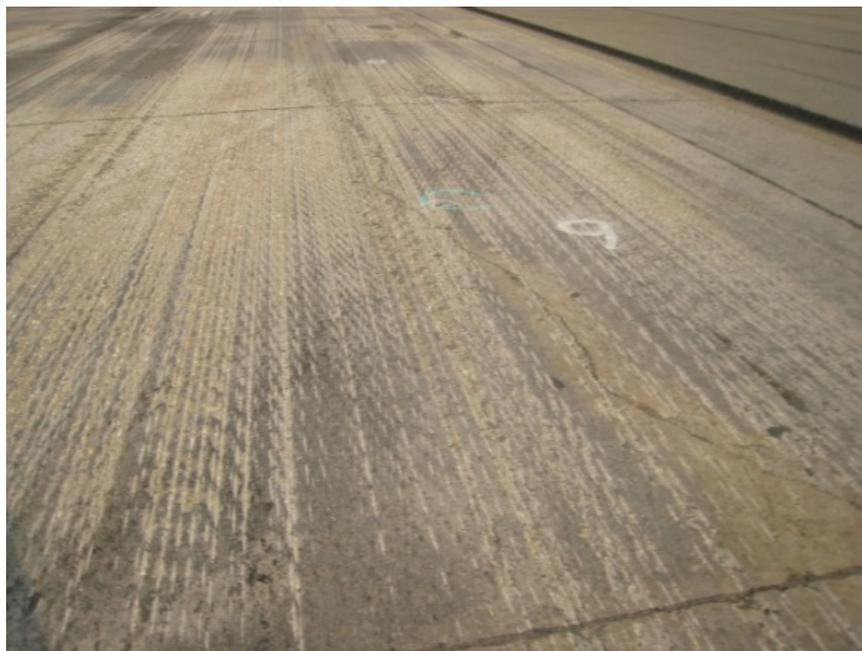
Photograph 6: Example of cross stitched crack in concrete slabs.
