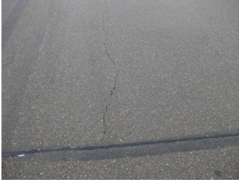
Photograph 2: Typical medium severity reflective cracking on the runway pavement.
