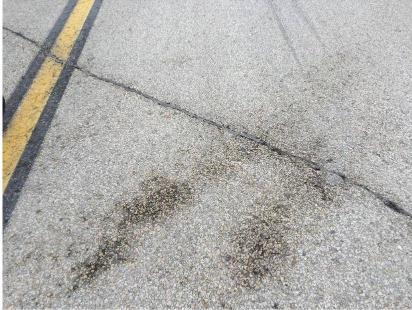
Photograph 13: Ravelling, cracking and polished aggregate.
