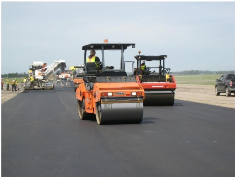
Photograph 9: Compaction operation on Runway 12-30.
