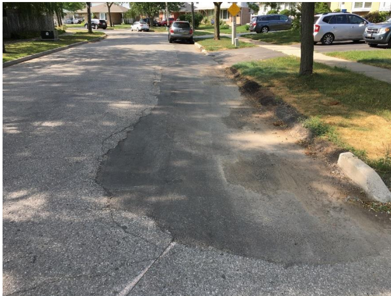
Photo 3: 1m Trench Restoration (Hand Laid), Altadena Court
