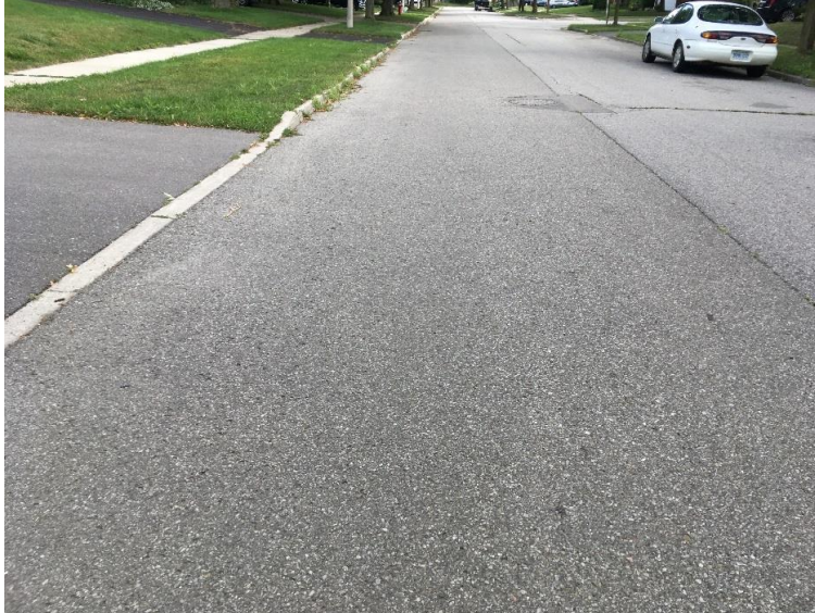
Photo 2: Typical 3m Trench Restoration, Sheridan Homelands
