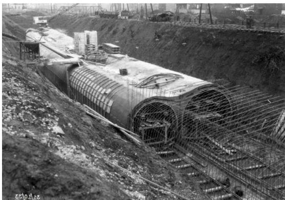
Figure 6. Construction of Collector Saint-Pierre
