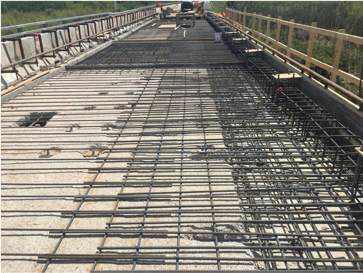
Figure 7 - New Top Mat Reinforcing of the Bridge Deck
