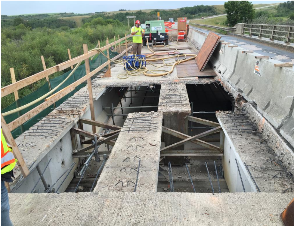
Figure 6 Demolition of the Deck at the Piers
