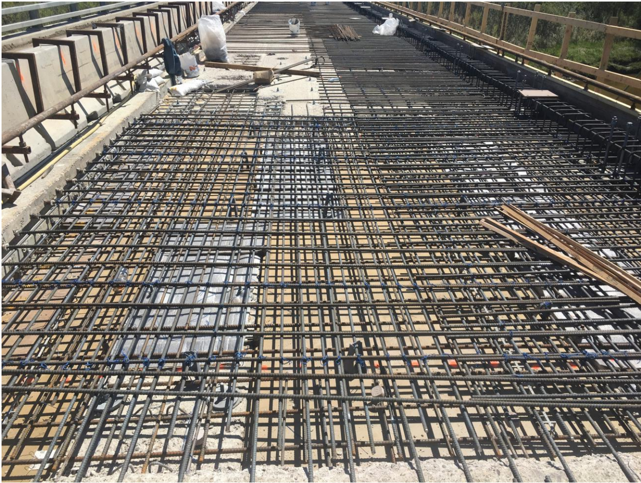
Figure 7 Link Slab Reinforcing
