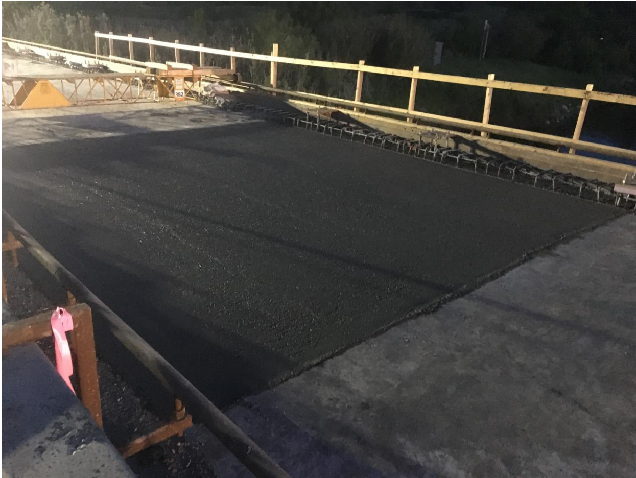
Figure 8 – Recently Placed Link Slab Concrete.
