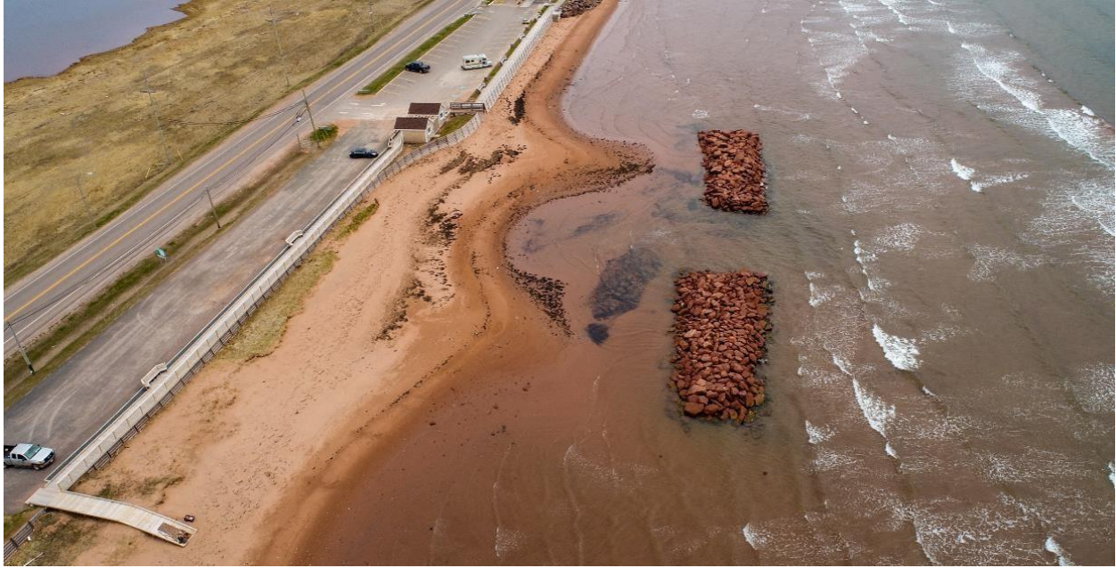
Figure 2 Oblique aerial April 2018
