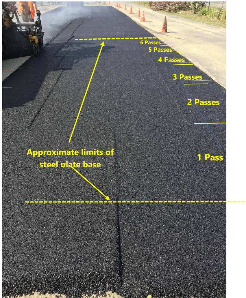
**Figure 1 – Roller marks indicating various compaction levels in trial section placed over steel plates.**
