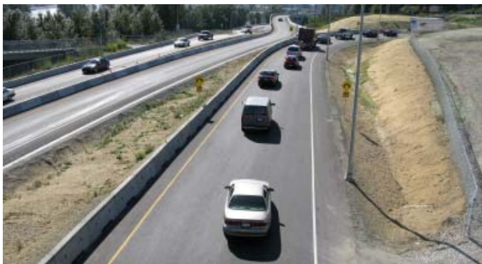
Photo: Geoffrey Ho, G. Ho Engineering Consultants Inc.
