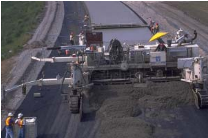
Photo: Dufferin Construction Company
