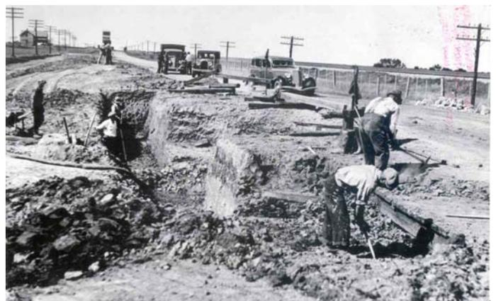
Excavating for rock drain and wooden drawing structure; Highway 2 Leduc to Millet (Alberta), July 1936. **Source:** Canadian Good Roads Association
