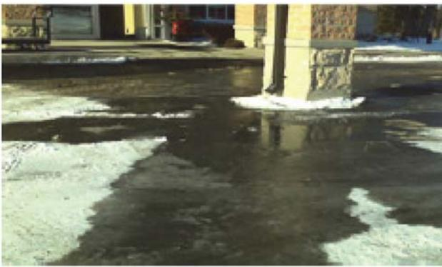
It is informative to view a site on a rainy day to understand how poorly designed facilities can affect drainage. The areas of poor drainage are clearly evident. These areas are prone to icing in cold weather and therefore are high risk areas for slips and falls and consequently become high salt use area. Effective drainage management can therefore reduce salt use over the life of the facility.
